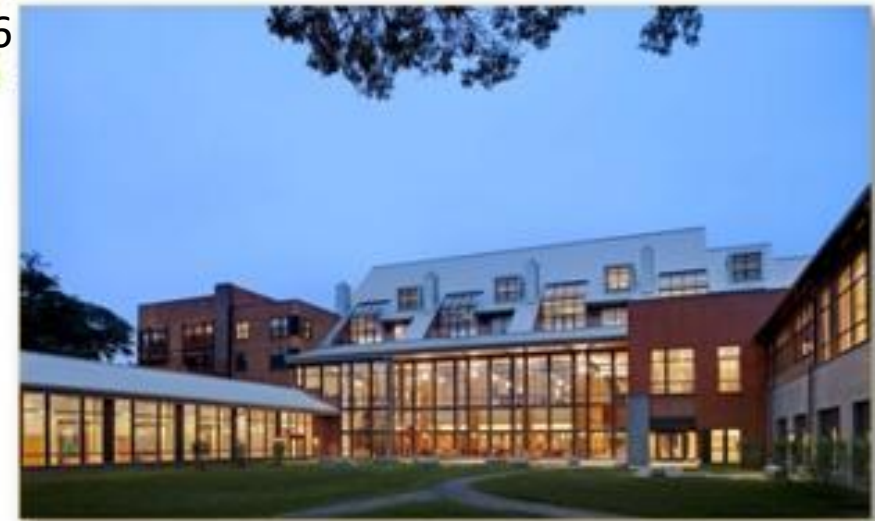
NewBridge on the Charles Dedham, MA
